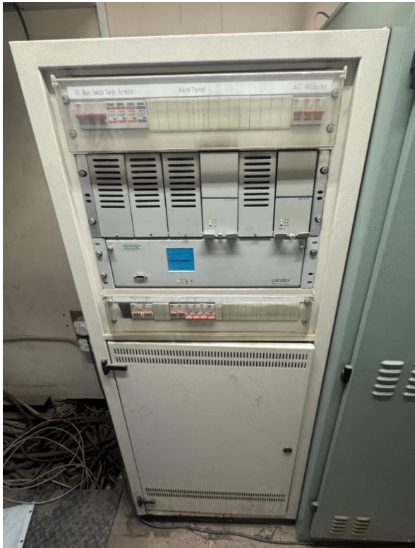
Figure A.7: NMC Charger for DC Loads
