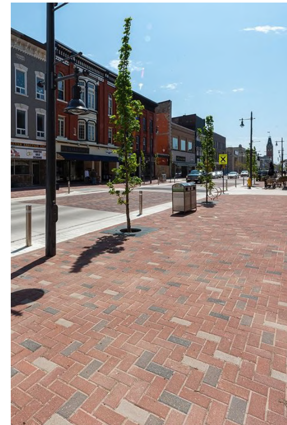
Wide sidewalk for NMT movement, street furniture and tree planting
