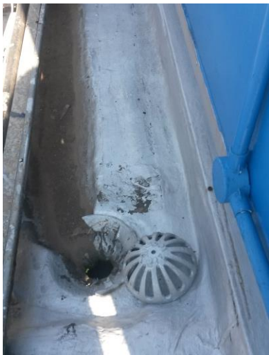
Figure 19: Condensate drains for Air Handling Units
