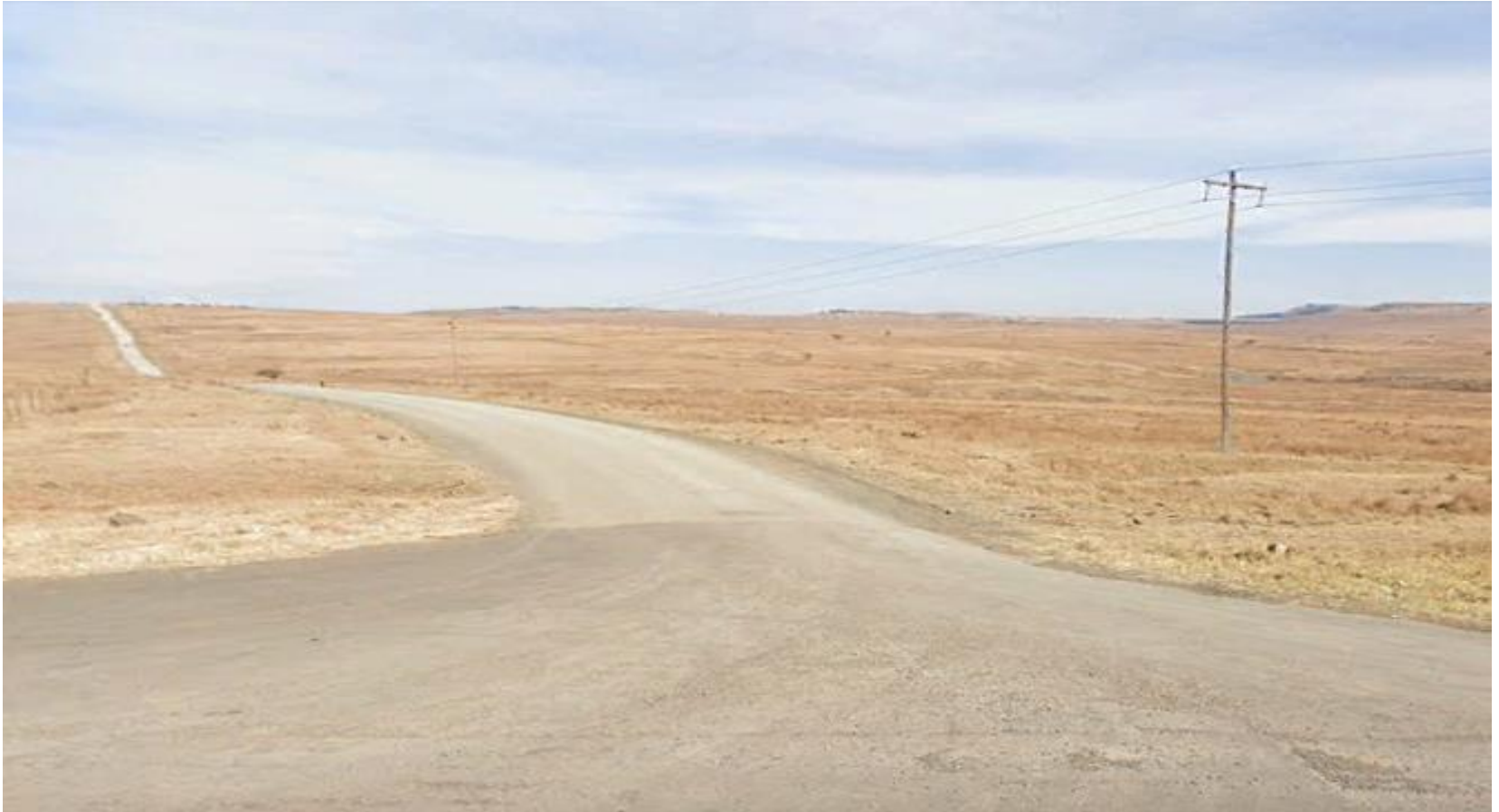
END OF PROJECT R68 & P372 Intersection (Ngwebeni Village) (Looking South West)
