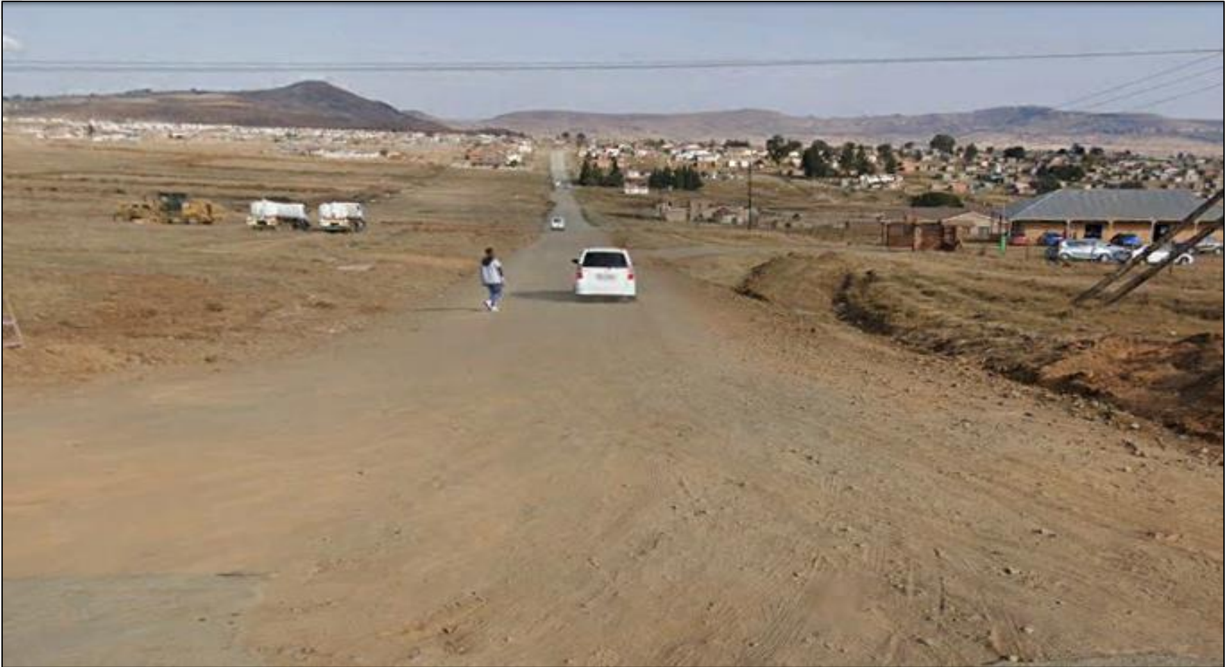
START OF PROJECT R68 & P372 Intersection (Luvisi Village) (Looking South)
