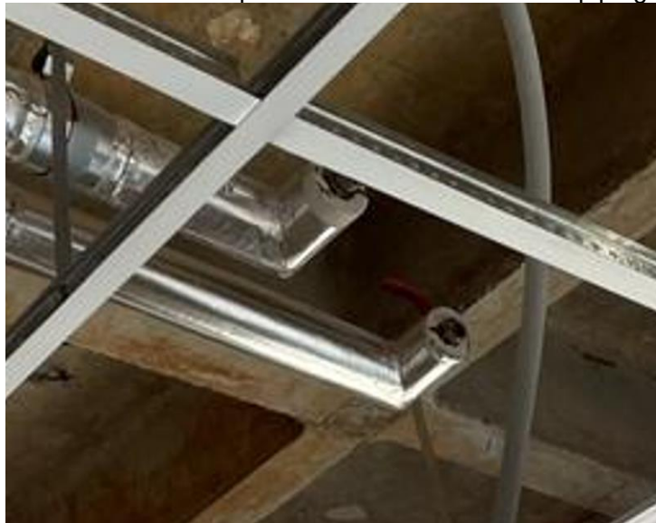
Figure 1: Chilled water connection point to FCU
