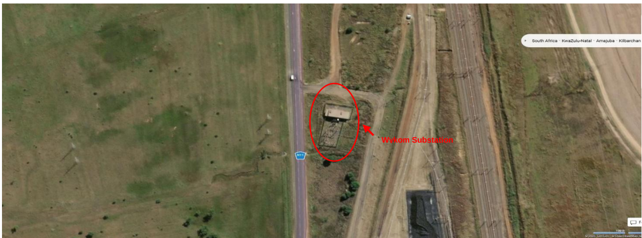
Picture 1: Wykom substation and surrounding Area (Main Road N11)
