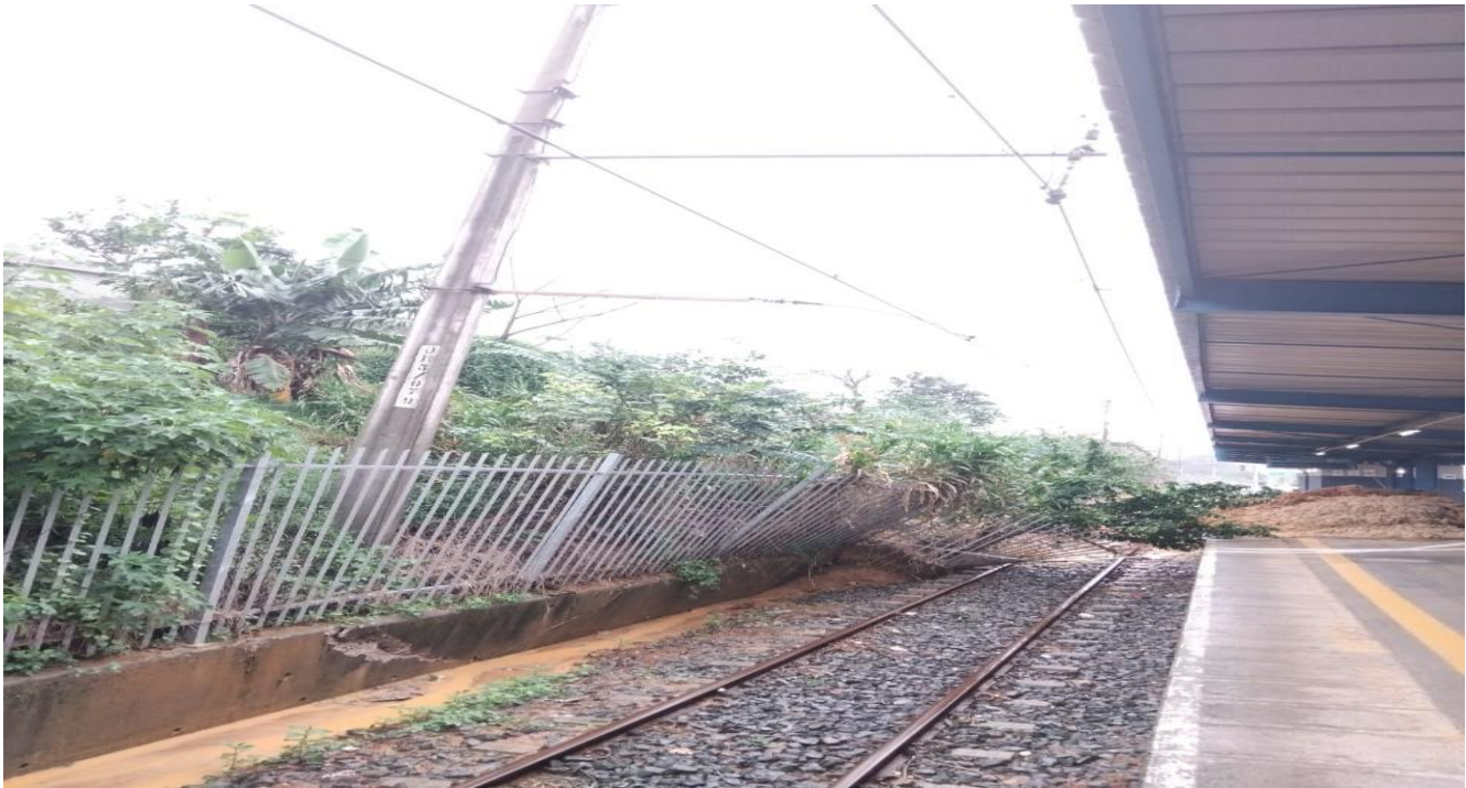
Figure: concrete mast pole
