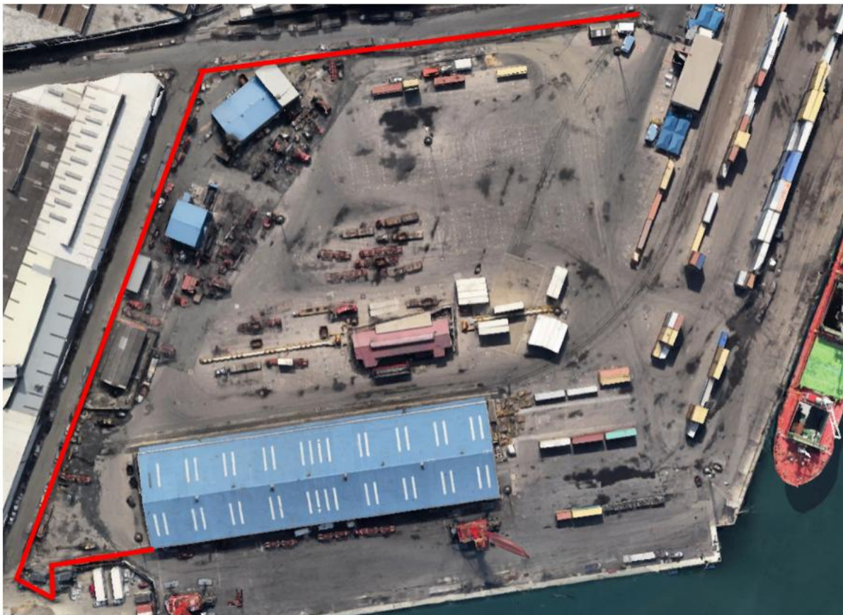
Figure 9: Maydon Wharf Berth 12
