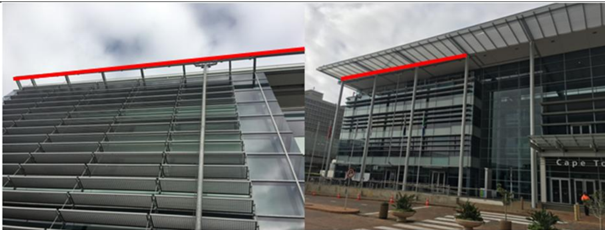
B3. NW Corner Monorails and trolleys
