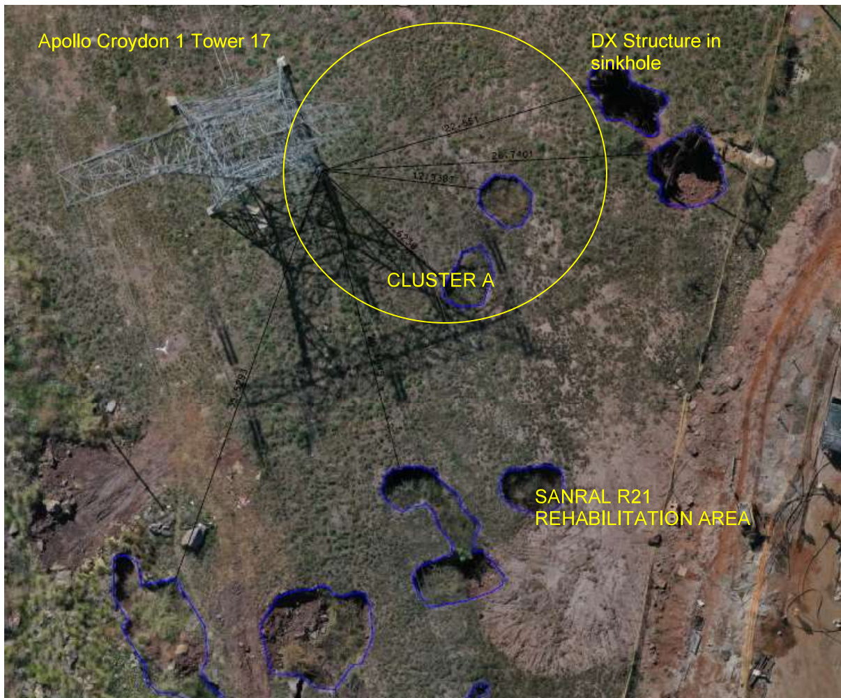
Figure 1-1. Apollo Croydon 1 275kV T17 R21: Annotated Locality Image
