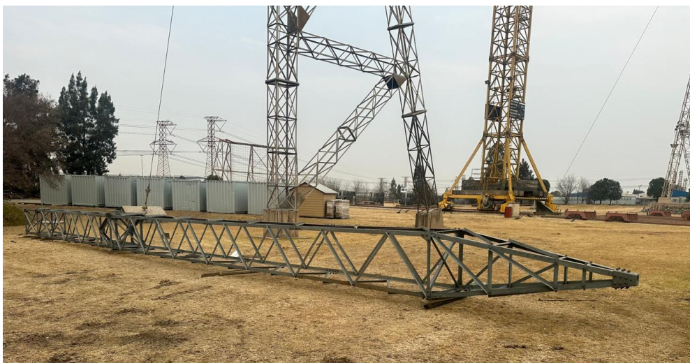
Figure 3: Actual structure to be used for practical evaluation
