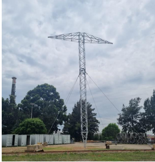
Figure 2: Type 704B structure
