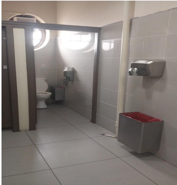
Figure 7 Female Toilet in Station Building with Toilet Roll holder, Waste Bin, Seat Sanitiser, SHE Bin, Hygiene Bag dispenser
