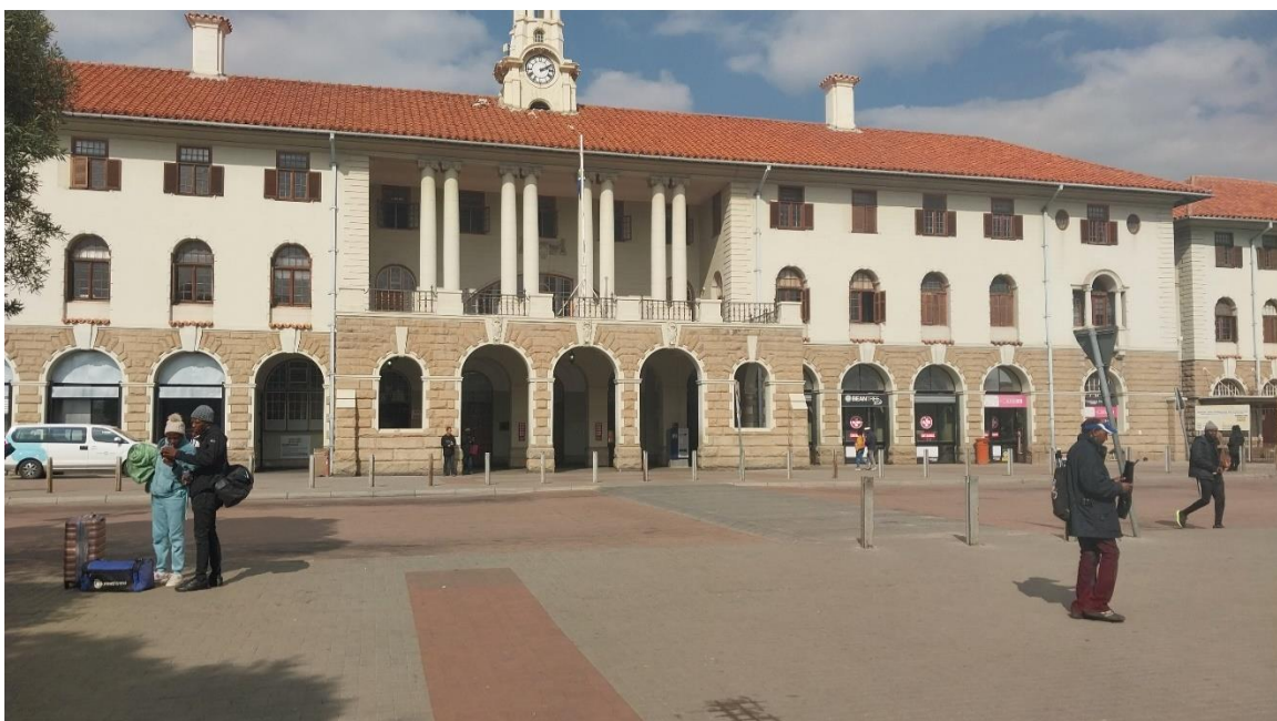
Figure 1 Pretoria Station Building
