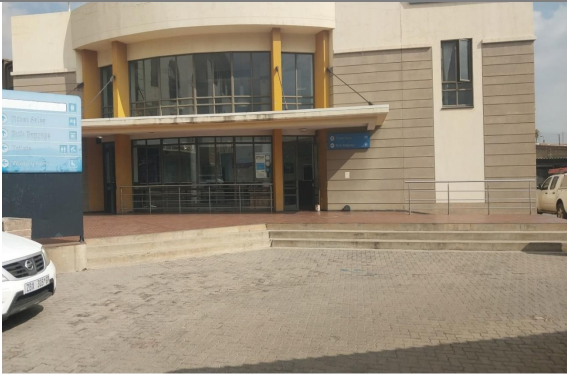
Figure 2 Shosholoza Meyl Building
