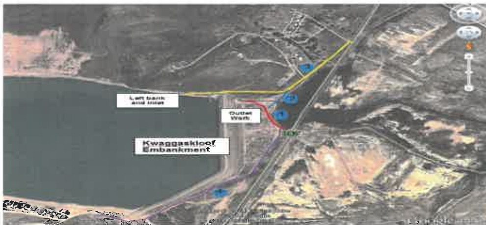
Figure 3: Plan view of Kwaggaskloof embankment (Google Earth, 2013)
