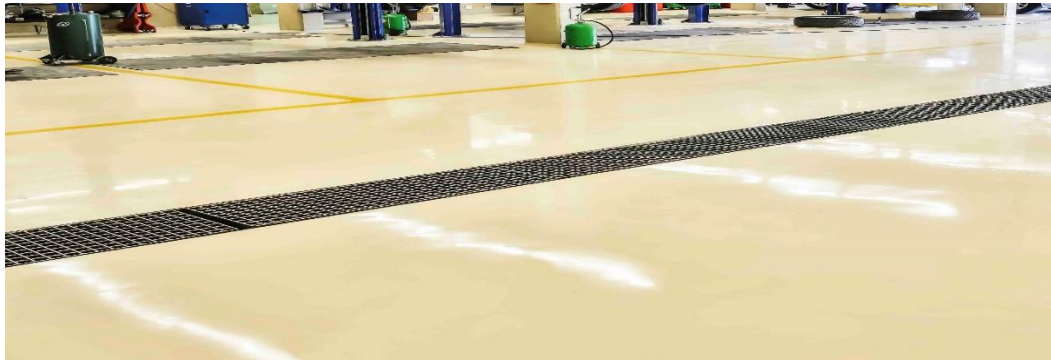
Example of epoxy floor
